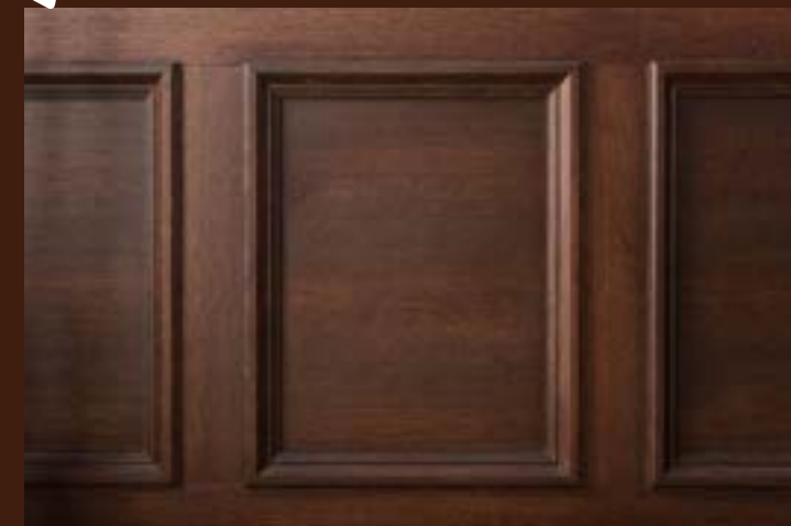
Wooden lower wall panels
